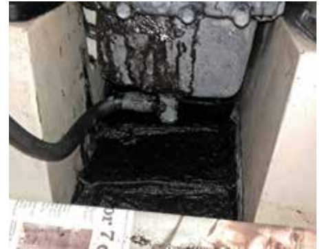
July Oil Leak
