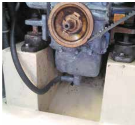
March Nice cleanup and paint job
