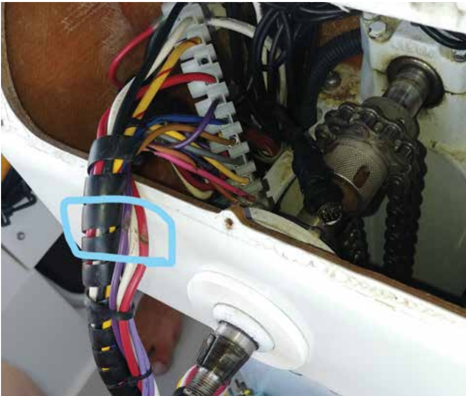
Chafed wires and steering chain
