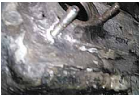
July dry fit before JB Weld
