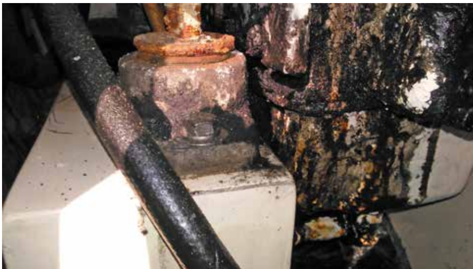
March First Oil Leak
