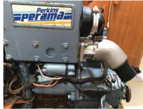
New elbow installed with new heat exchanger boot and black 1-3/4" to 2" adapter in place.
